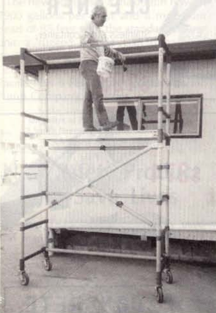
Erection of this lightweight structure took only a few minutes and immediately provided this tradesman with a safe and effective work platform in new Fiber-Tek.
